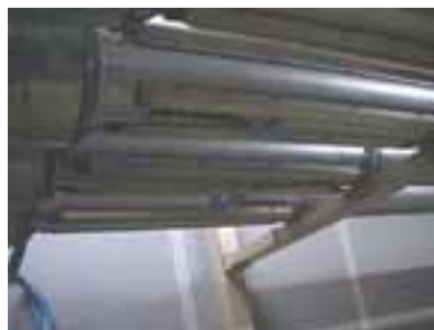
Clear Tubes installed
