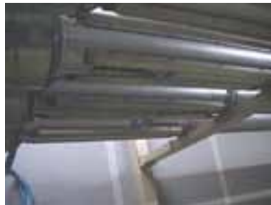
Clear Tube installati
